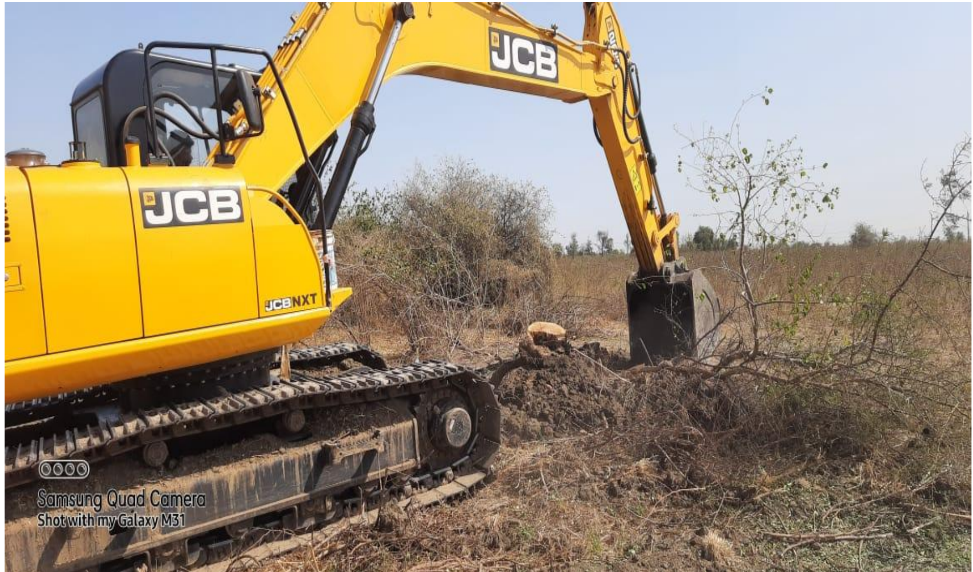
C&G work and Roots removal in progress
