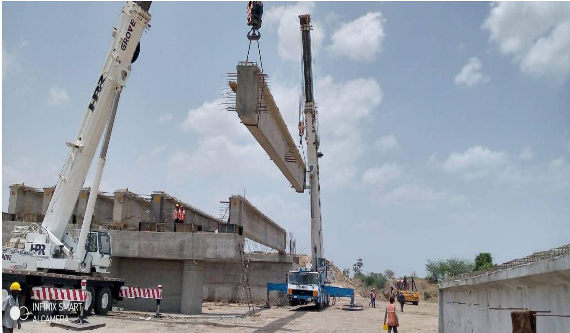
Girder launching at Major Bridge Ch-359+936
