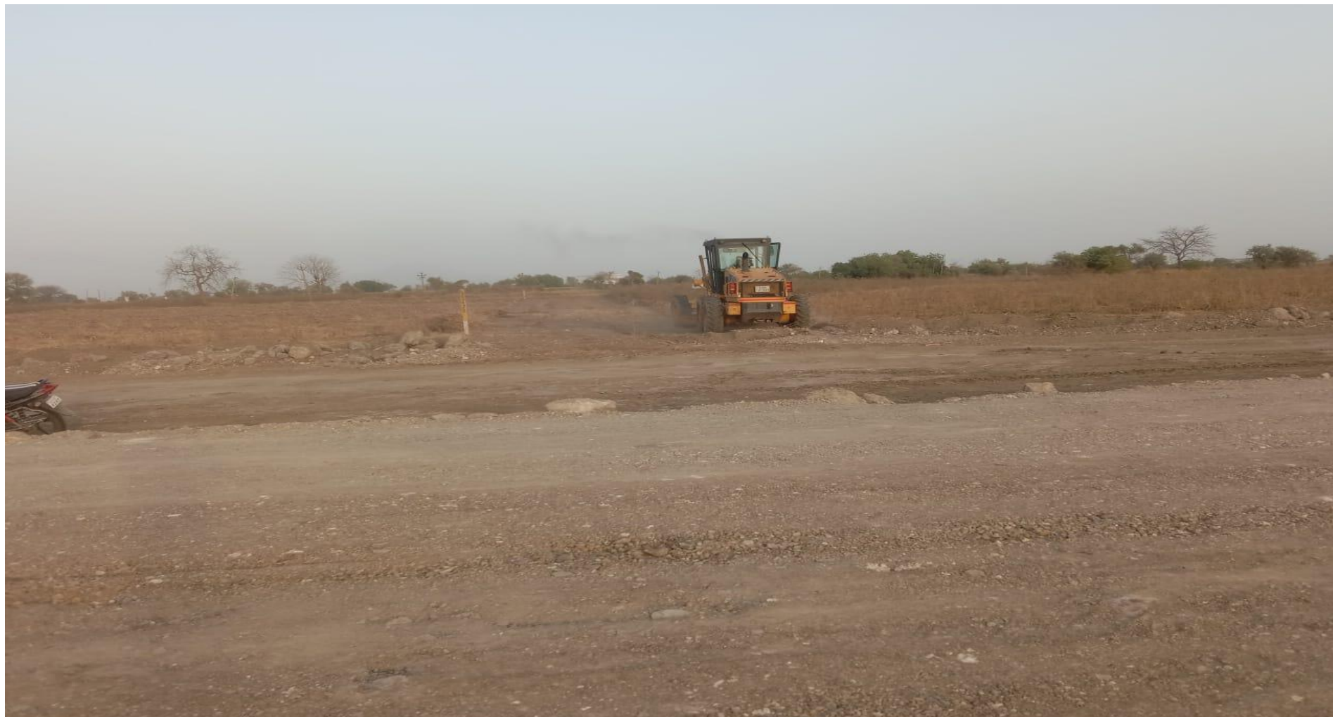
Cleaning and Grubbing wor progress at project site
