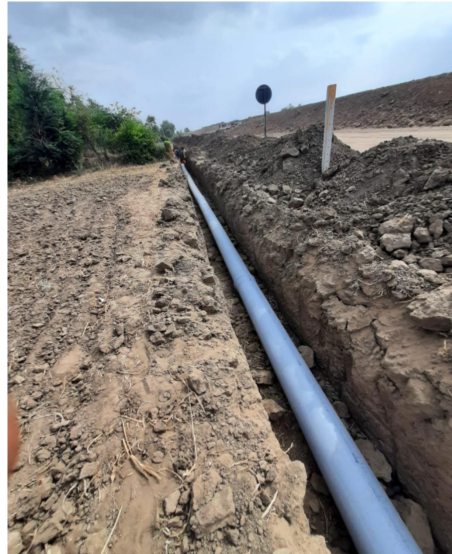
UGPL pipe laying work in progress 356+700 rhs
