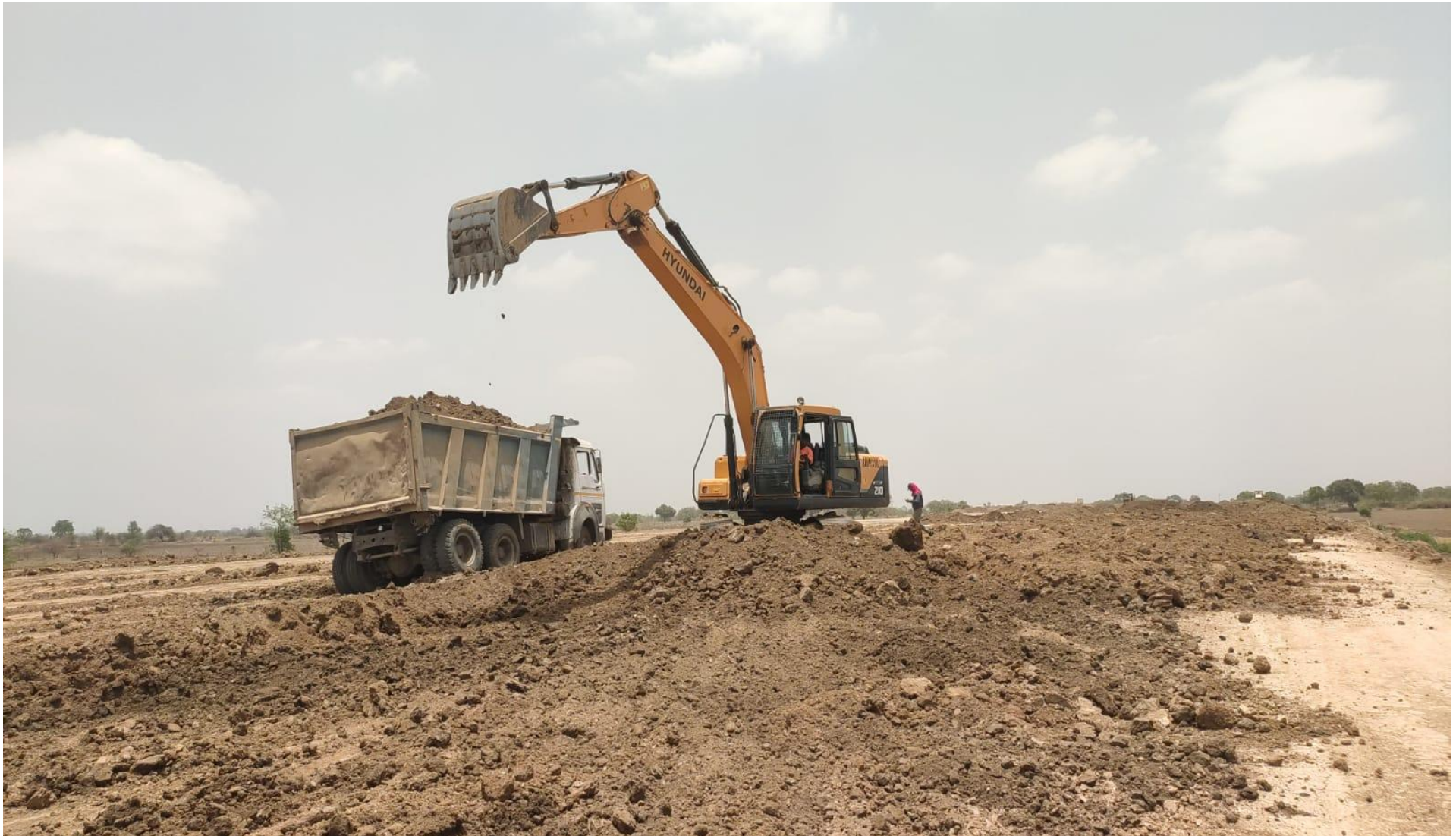
Black cotton soil removing at site
