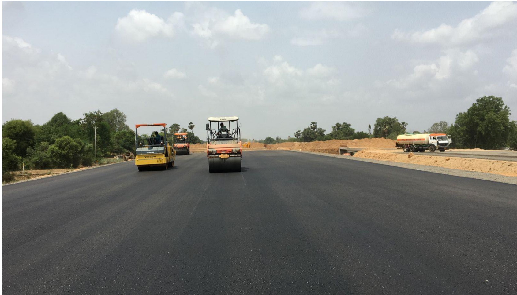
DBM-1st Rolling In Progress
