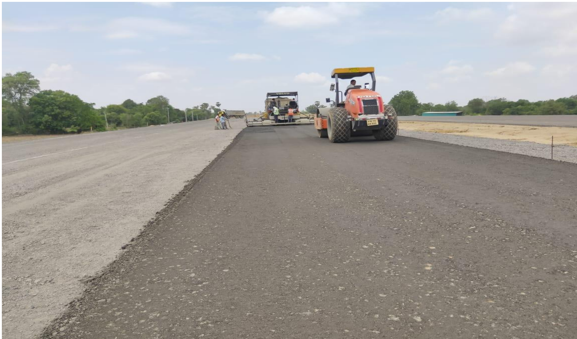
WMM laying in progress
