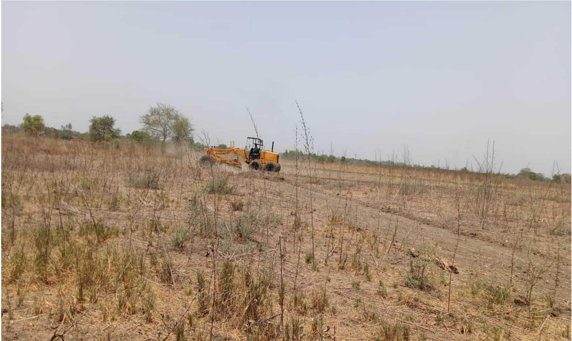
C&G work in progress at ch.363+310
