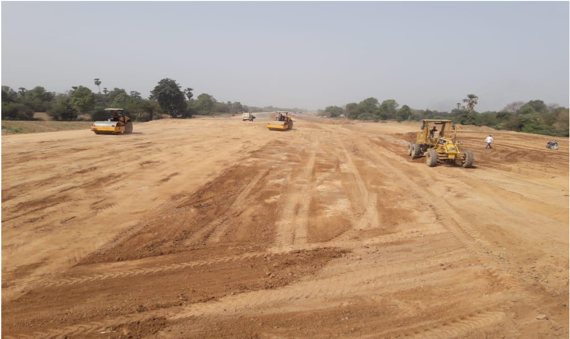
Embankment Layer in progress
